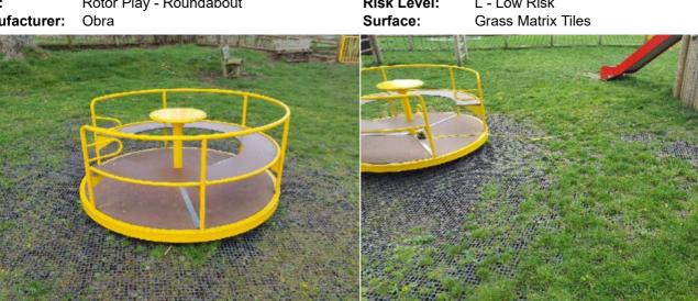
Finding: The falling space overlaps the free space between Action: Monitor - No remedial work recommended the roundabout and the tunnel mound / embankment slide in contravention of the requirements of BS EN 1176:2017 Part 1
