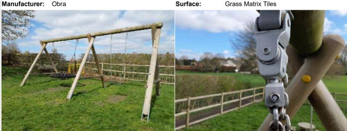
Finding: The swivel joint is worn and requires replacement Action: Replace
