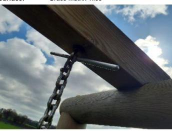
**Finding:** The connecting links are in excess of 8.6mm and less than 12mm and fail the requirements of BS EN 1176 Part 1; clause 4.2.13, Chains
